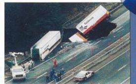
abnormally heavy rains in November undermine the roadbed of Oregon's Interstate 5, creating a 40-footdeep sinkhole, into which two semitrailer trucks tumble.
